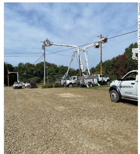
BUCKETS BRIGADE: Four buckets with journeyman lineworkers build out lines to a new member's service location.
