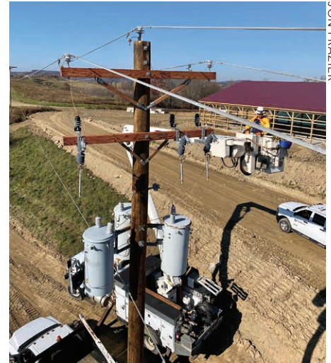
THE POWER BEHIND YOUR POWER: Journeyman Lineman Jordan Stear prepares to install this three-phase service in Punxsutawney.
