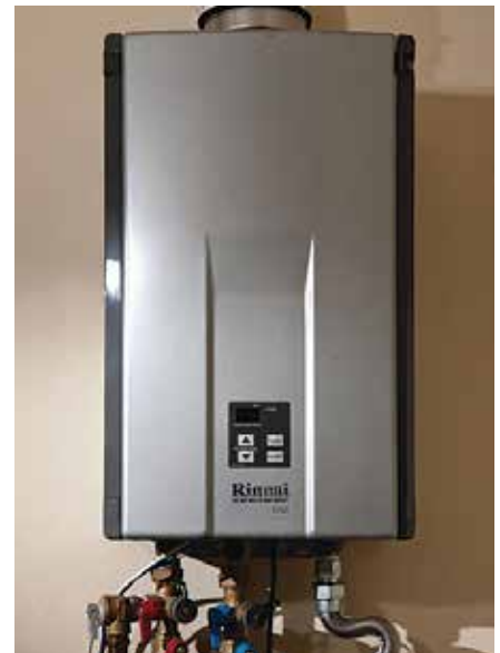
A SAVINGS?: Electric tankless units only use energy when someone needs hot water, which sounds great, right? The problem is, tankless systems require a great amount of energy to heat water quickly.
