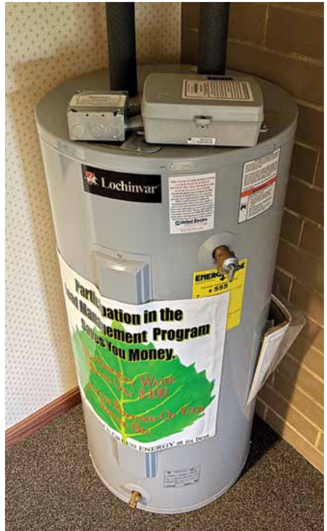
LOAD MANAGEMENT: This standard electric hot water tank is equipped with a demand response unit, which helps United Electric and its members better manage peak demand periods during the summer.
