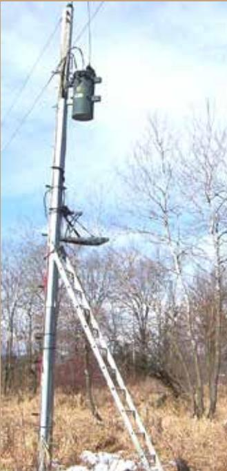
Lineworkers climb poles at all hours, in the worst conditions. Sharp objects like nails, tacks or staples can puncture our rubber safety equipment, leading to electrocution. While climbing, lineworkers use small spikes, or hooks, to grip the wood of the pole. One misplaced hook caught on a nail or staple will result in serious injury to our lineworkers.
