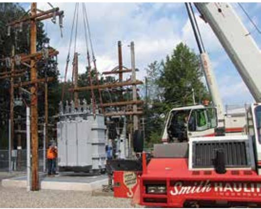
**PLACING TRANSFORMER:** Smith Hauling, one of United Electric's members in the Ringold area, places the new 5-MVA transformer in the new Robertsville Substation.
