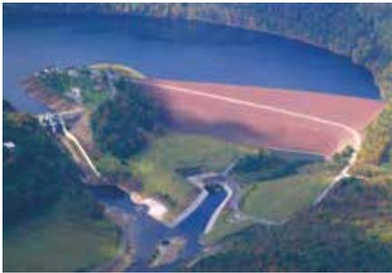
**POWER SUPPLY:** The William F. Matson Generating Station, a 21-megawatt generation facility at the base of the Raystown Dam, provides enough power to supply 8,500 Pennsylvania co-op members' homes.
