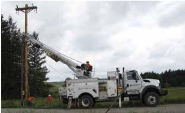
**SETTING POLE:** United Electric linemen Jason Duttry, Jayme Good and Dan Marshall set a pole near Sprankle Mills Road. This pole is part of the Oliveburg line upgrade that will allow us to backfeed the Grange, Robertsville and Conifer substations.
