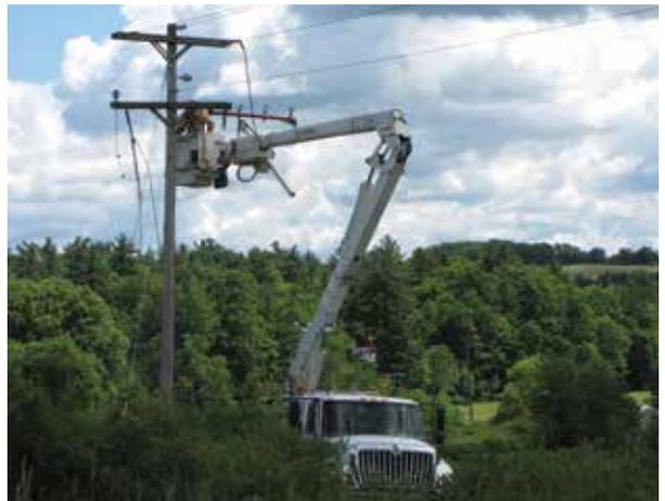
**REMOVING LINE:** United Electric linemen remove small capacity copper wire to make way for an upgrade to a larger capacity conductor in the Oliveburg area.
